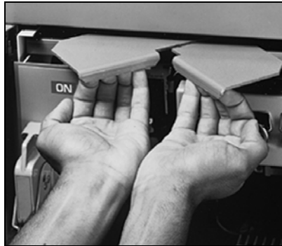
Figure 66: Pulling the Twin Handles of the Cam Mechanism Forward
