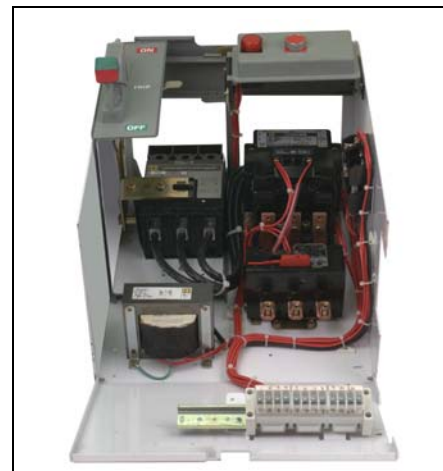
8998-9853 Figure 47: Control Unit Bottom Plate Folded Down
