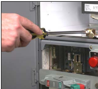
Figure 68: Tightening the Control Unit Lock-in Device (when supplied)
