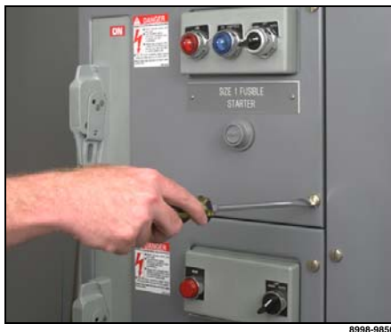
Figure 39: Loosening Captive Quarter-turn Fasteners
