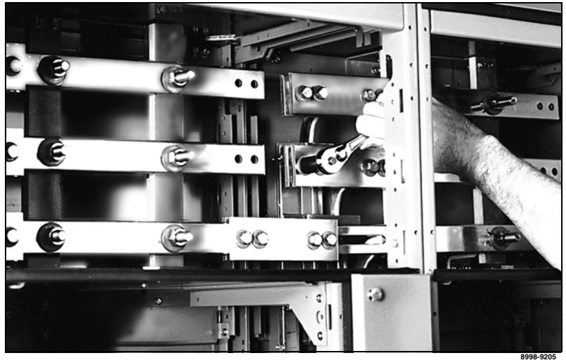
Figure 17: Removing the Left Bolts and Loosening the Right Bolts on the Splice Assembly
