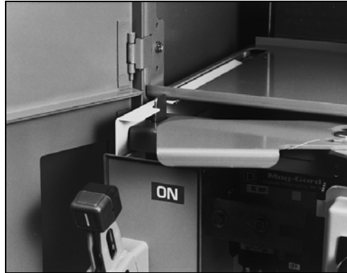
8998-9218 Figure 44: Operating the Mechanism-to-Structure Interlock
