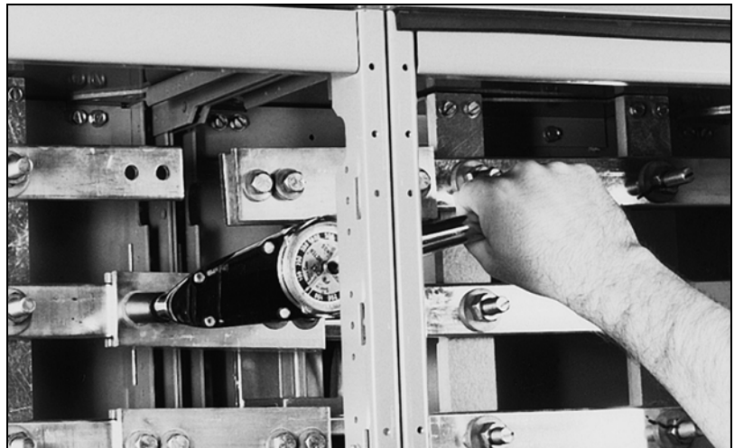
Figure 20: Torquing the Bolts
