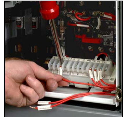
Figure 70: Connecting Control Leads to the Terminal Blocks
