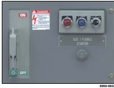
Figure 38: Operating Mechanism in the Off Position
