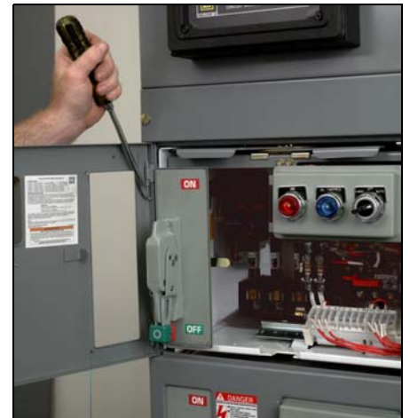
8998-9941 Figure 48: Driving Out Hinge Pin
