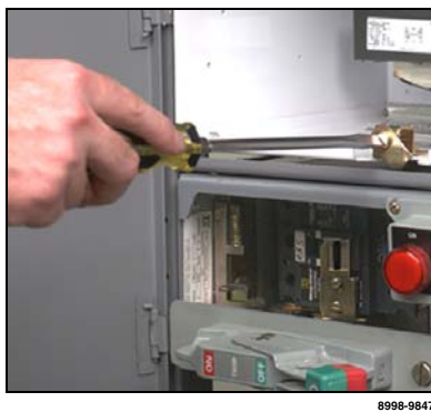
Figure 40: Releasing the Lock-in Device (when supplied)
