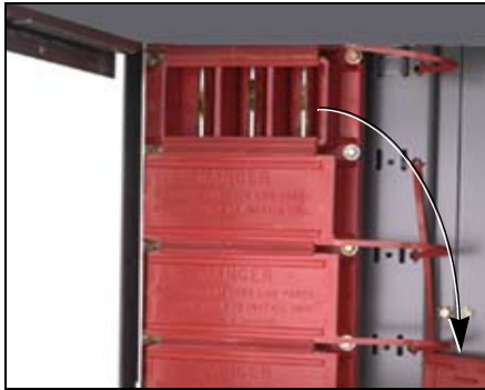
Figure 65: Removing the Manual Bus Shutter
