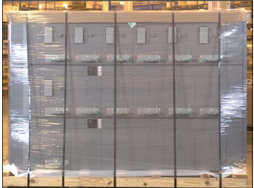
Figure 1: Packaged Motor Control Center
