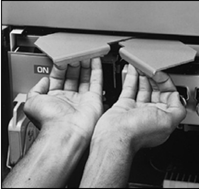
8998-9249 Figure 43: Pulling the Twin Handle Cam Mechanism Forward
