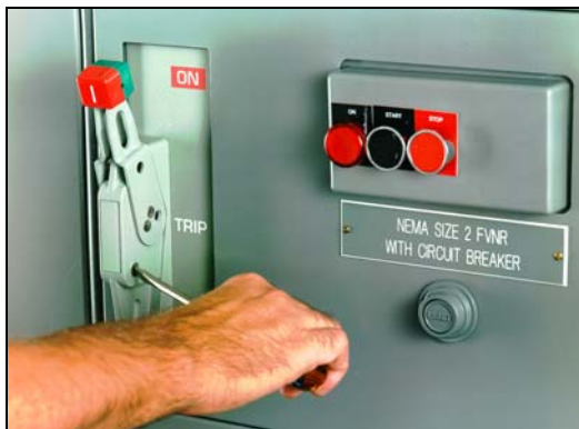
Figure 61: Operating Door Interlock Defeat Mechanism
