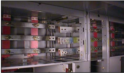
Figure 21: Bus Covers Removed
