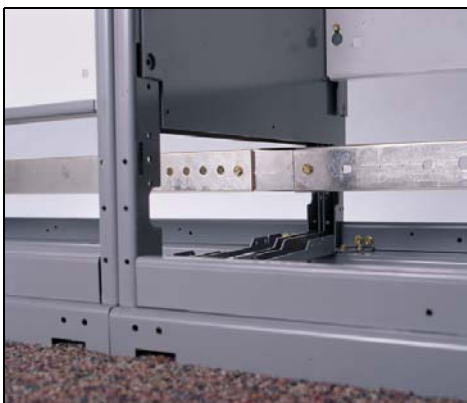
Figure 27: Ground Bar Bolt Replaced
